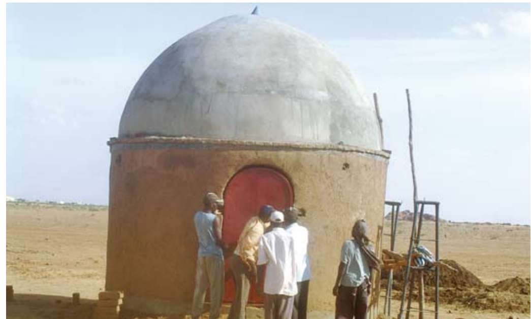
Pic 28. A completed dome roof house model
