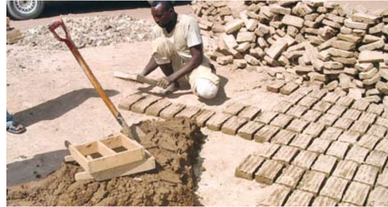
Pic 4. A participant using a moulding cast for brick production
