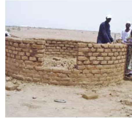
Pic 7. The wall is built up leaving a gap for the door
