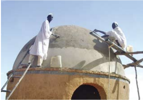
Pic 22. Plastering the roof.
