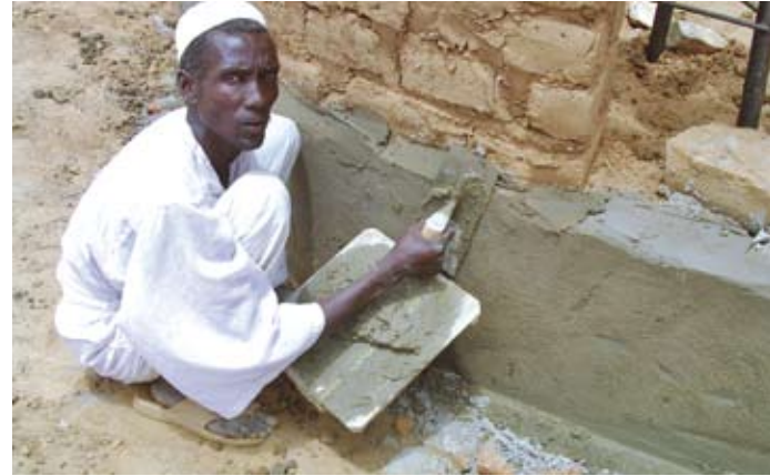
Pic 13. Plastering the base of the house
