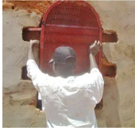
Pic 26. The window frame is inserted
