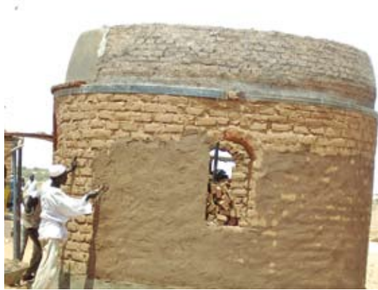
Pic 23. Plastering the outer walls
