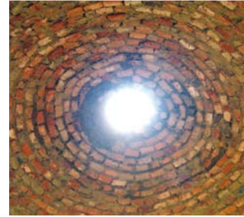
Pic 20. The dome roof from inside, a small hole is left in the top for ventilation
