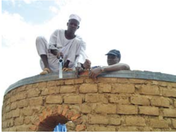
Pic 12. Using the steel clamp to support the walls
