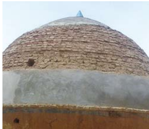
Pic 21. The metal hole cover can just be seen at the top of the house
