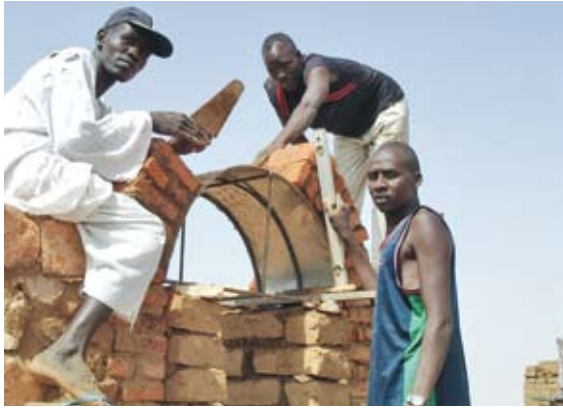
Pic 8. Building the window arch using a metal girder
