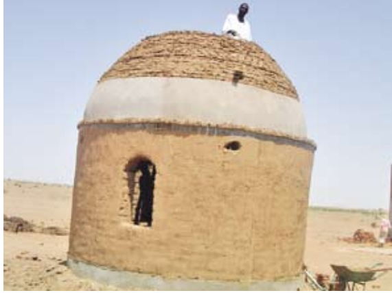
Pic 19. Further courses are added to form the dome
