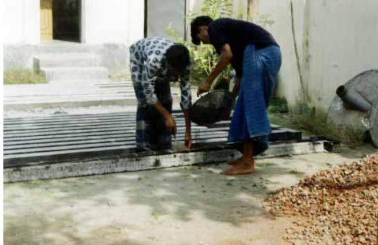
Figure2 Construction of RCC pillars by Bandhan Society
