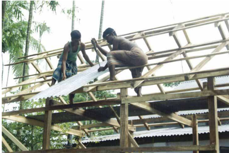
Figure 3 Construction of a rural house in Kishoregonj, Bangladesh
