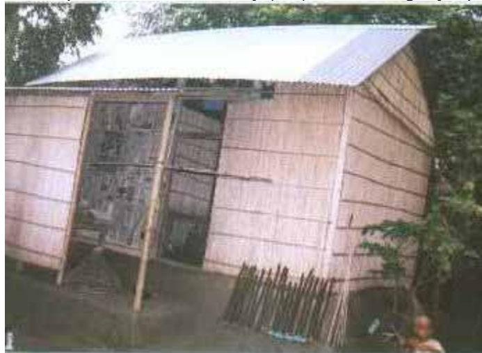
Figure1 Village house with raised platform demonstrated by ITDG Bangladesh
