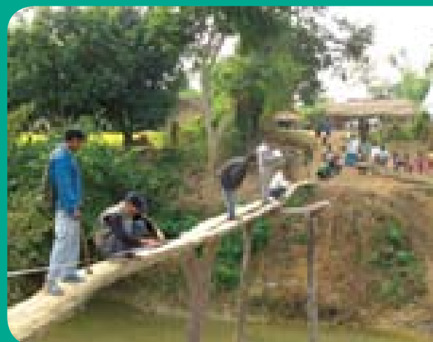
Wooden logs were used to cross Kanjarawa Nala before the bridge construction
