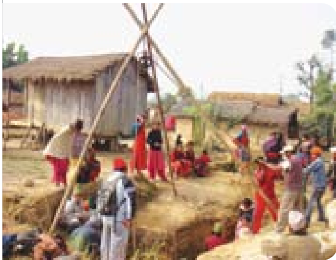
Communities working together to install shallow tube well
