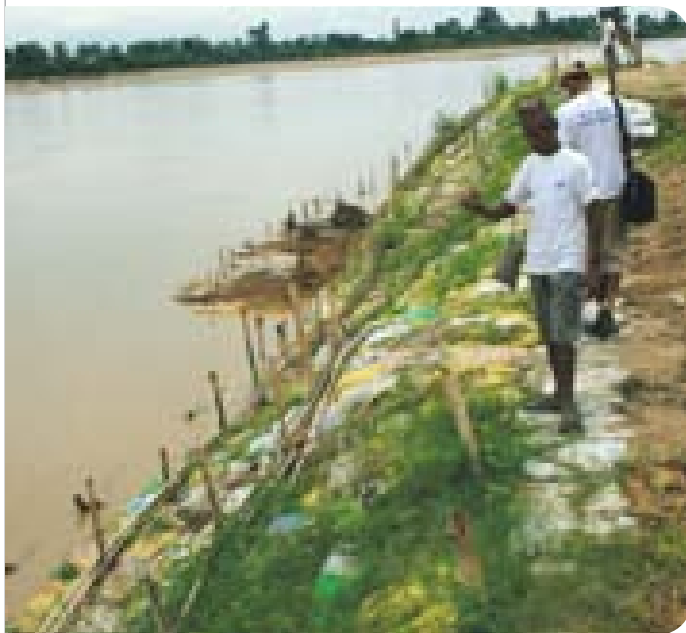
Application of bio-engineering technique to strengthen Babai river banks
