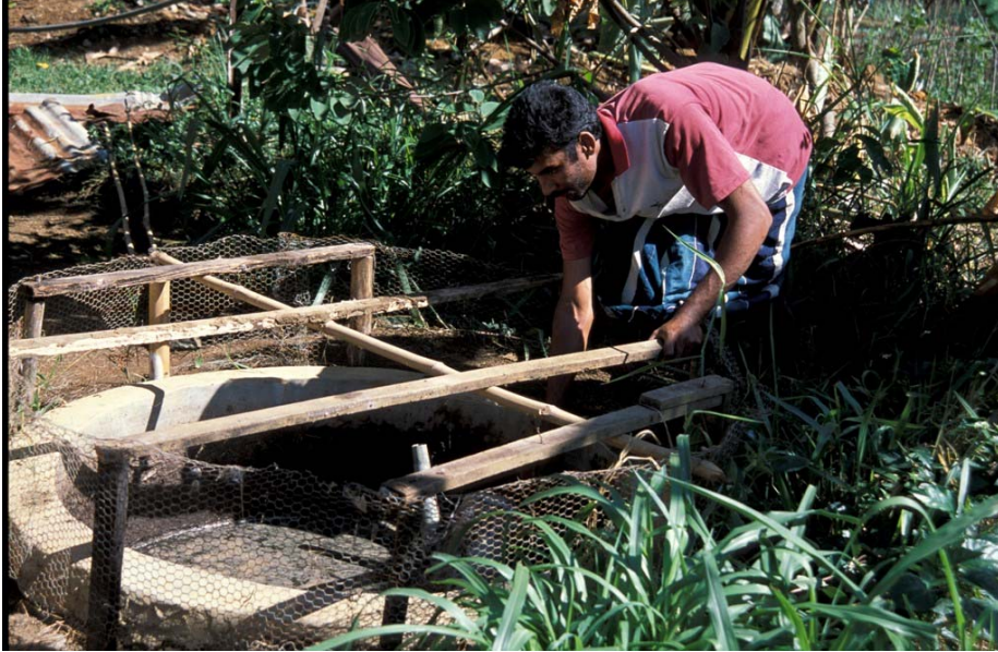
Bio-digester from a plant in Sri Lanka
