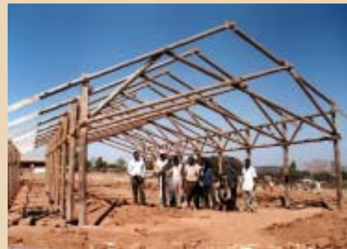
Timber pole framework for school building in Malawi. Photo by TRADA
