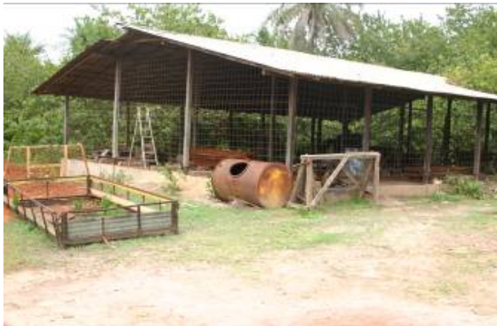
Photo 14 - Storage facilities SBI UPAA
