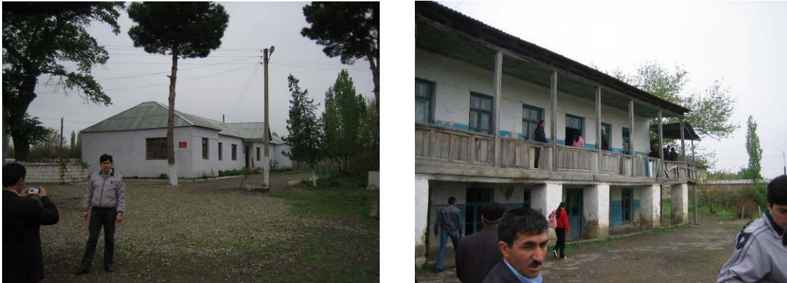
Figure 21 - Gimli Boluslu School newest building (left) and oldest building (right)
