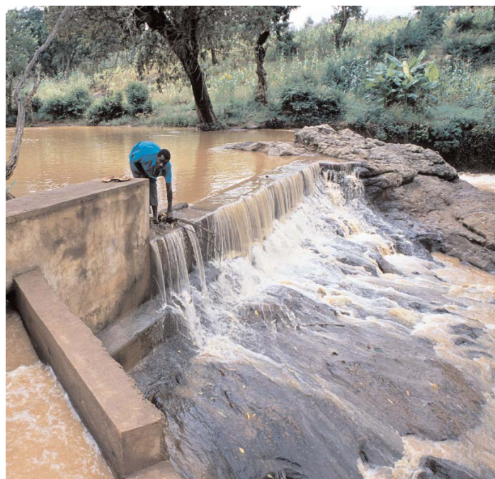
A micro-hydropower scheme supplies energy to light homes in a Kenyan village.
