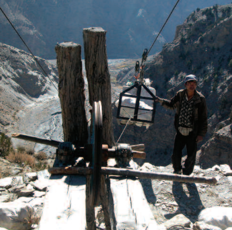
Goods being transported to the upper station of the gravity ropeway
